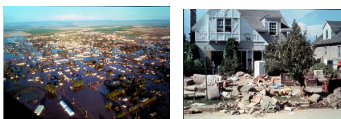
Figure 5: Damages due to Teton dam failure
