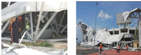
Figure 4: Damages due to SMZA collapse
