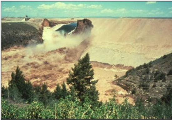
Figure 2: Teton dam failure
