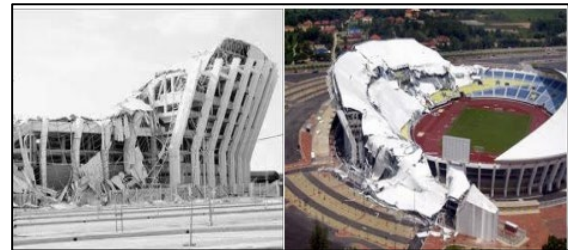
Figure 1: SMZA stadium collapse
