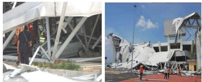
Figure 4: Damages in SMZA collapse
