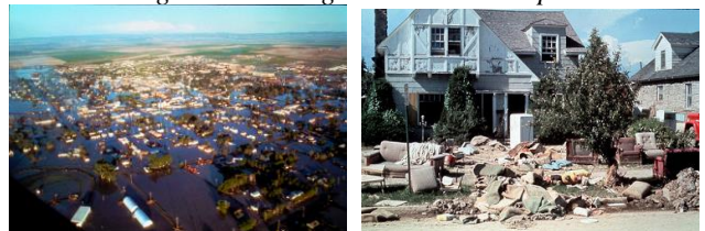
Figure 5: Damages in Teton Dam's failure causes flood to few towns
