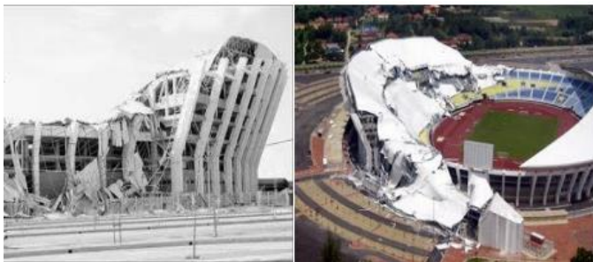
Figure 1: Stadium Sultan Mizan Abdidin collapse
