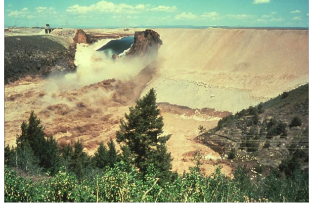
Figure 2: Teton Dam's failure
