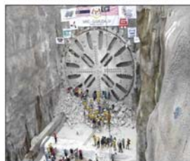
TBM TUNNEL – SOUTH DRIVE
