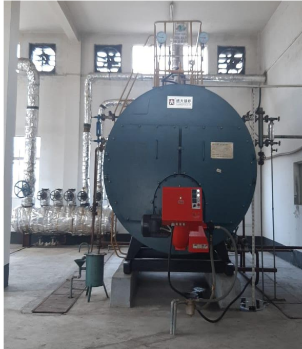
Figure 4.2.5.2 Diesel Boiler
