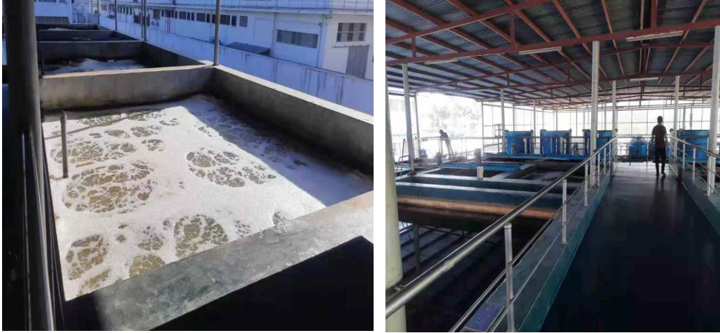
Figure 4.2.4.1 Coagulation and Sedimentation Tanks of WTP
