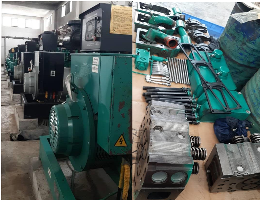
Figure 4.2.3.1 Cummins Generator KTAA19-G6/G7 Parts Disassembled
